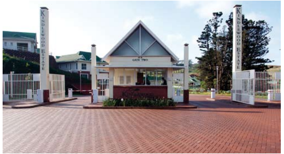
Kindlewood Estate entrance at Gate Two. All the roads in this development have been paved with Corobrik 60 mm burgundy pavers, laid in a herringbone pattern. Sidewalks have been paved with Corobrik 50 mm burgundy pavers.
