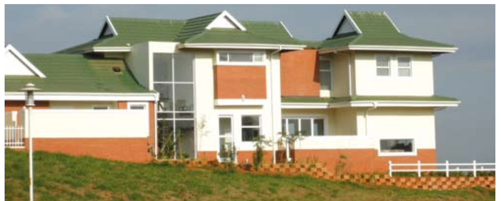
Corobrik clay facebricks were also specified at Kindlewood Estate, for plinths and feature walls on all buildings.
